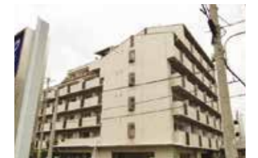
KGU International Residence III (西宮市)
